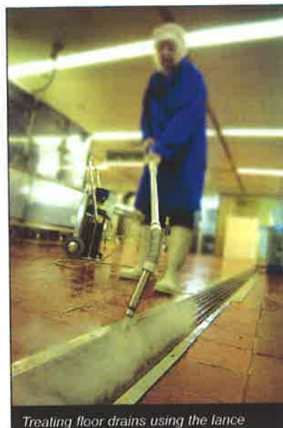
Treating floor drains using the lance
